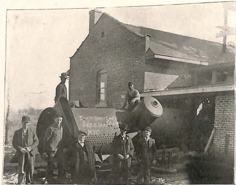
PUTTING ONE OF THE BIG BOILERS IN THE NEW HEATING PLANT.
